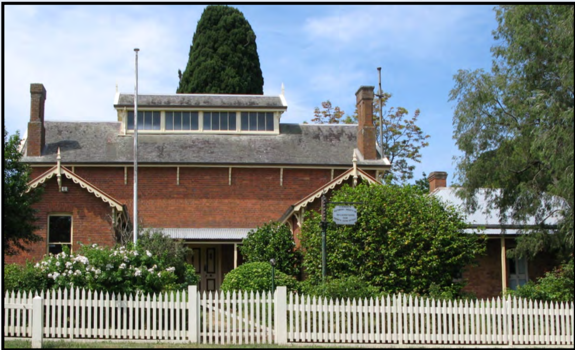
The Old Shire Offices, 326 High Street, Learmonth, Victoria.
